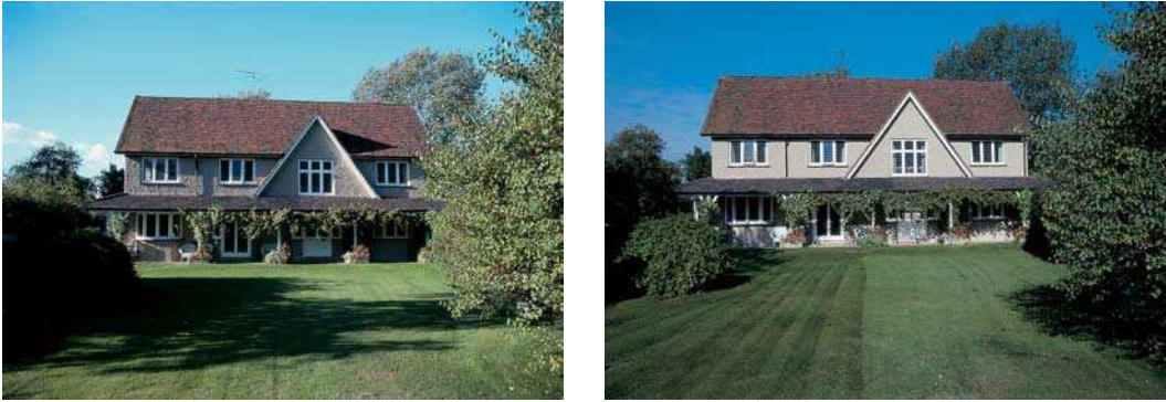
Figure 18.3 A building's texture, pattern and form change appearance as the sun moves direction during the day.
